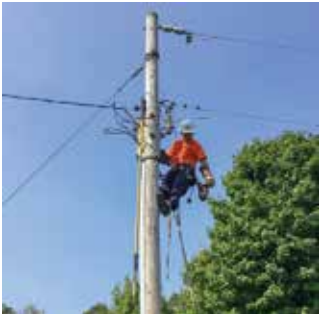
Dennis Vollrath, Polk-Burnett lineworker for 53 years
