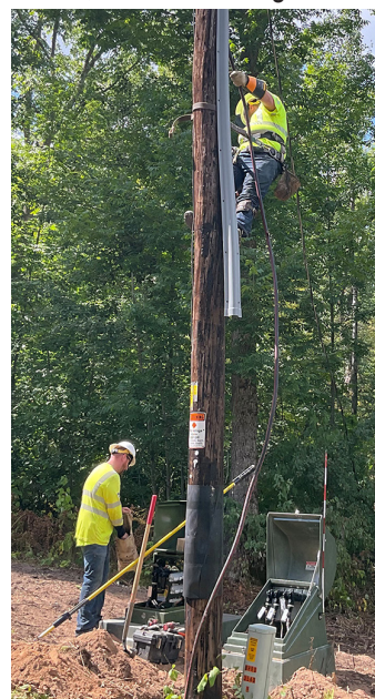
The co-op invested $5 million into grid upgrades in 2026. Our work plan includes converting miles of power line from overhead to underground to improve your reliability.
